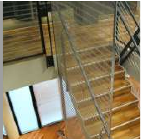
* Typical Architectural Installation
