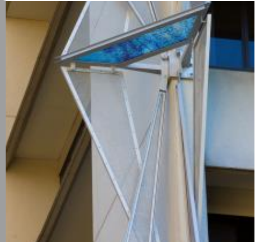
* Typical Architectural Installation
