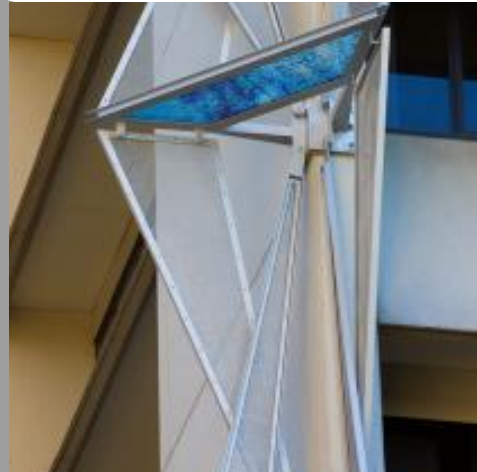
* Typical Architectural Installation
