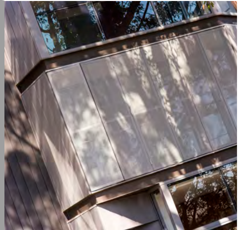
* Typical Architectural Installation
