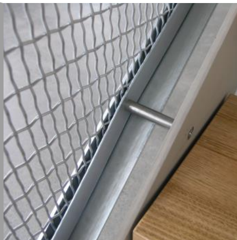
* Typical Architectural Installation
