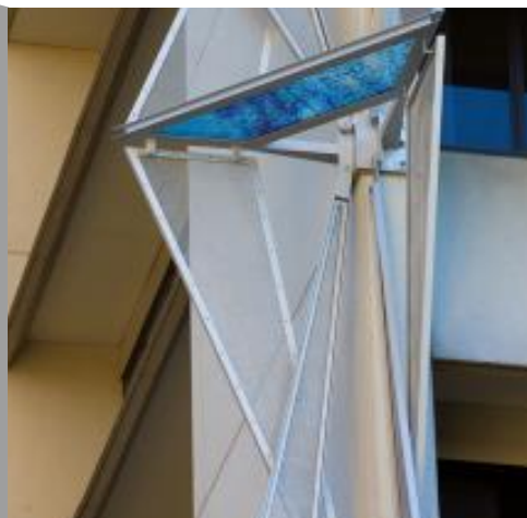
* Typical Architectural Installation
