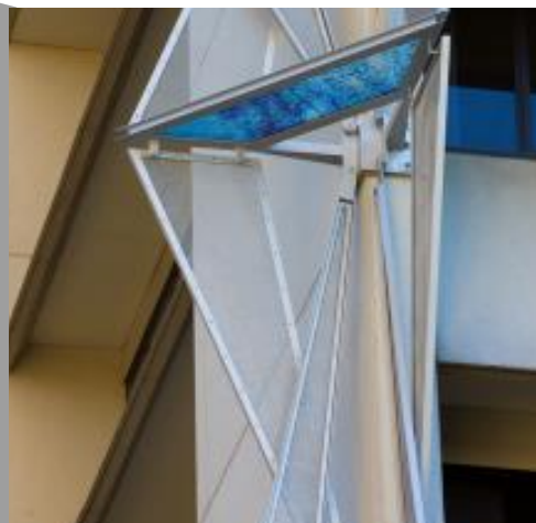
* Typical Architectural Installation
