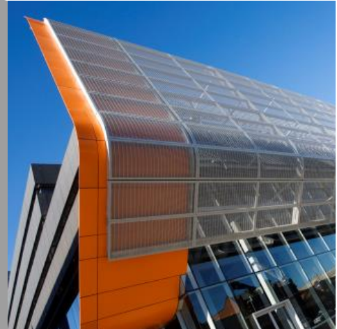
*Typical Architectural Installation
