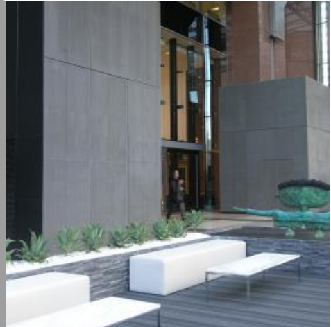
* Typical Architectural Installation
