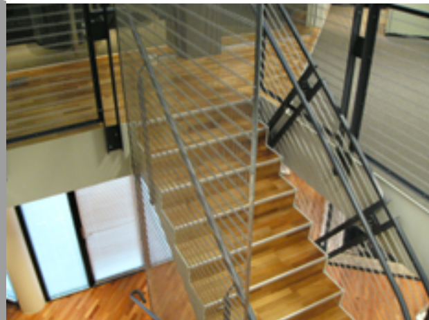
* Typical Architectural Installation
