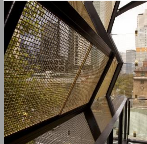
* Typical Architectural Installation
